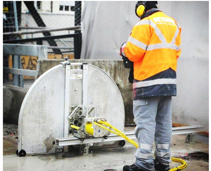
Concrete Cutting: 16KW, 9,000 RPM
