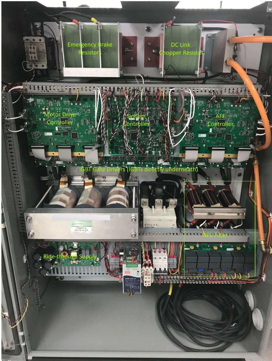
**Figure 35: Complete Beta/Gamma MLI Controller in IPC52 Cabinet**
